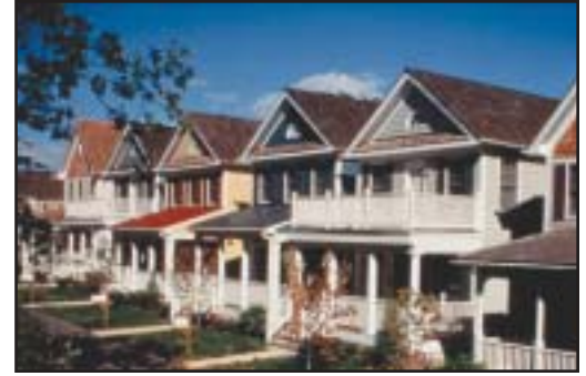
11 to 15 units per acre Kentlands, Gaithersburg, Maryland
